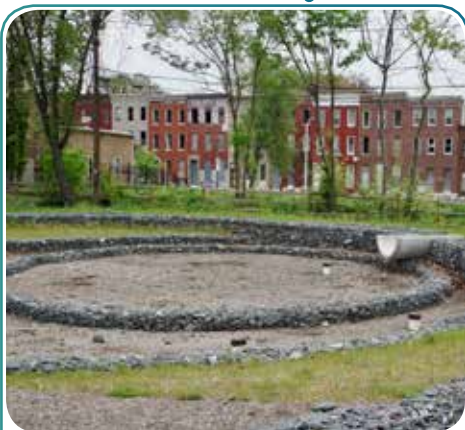
Type: Bioretention and asphalt removal Location: Harlem Park Project by: Baltimore City DPW
