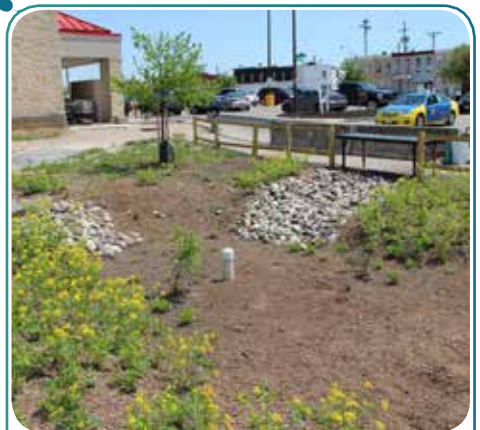
Type: Bioretention/rain garden Location: Highlandtown Project by: Blue Water Baltimore
