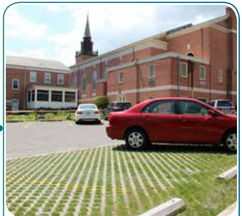
Type: Asphalt replacement and bioretention Location: St. Anthony of Padua Project by: Blue Water Baltimore
